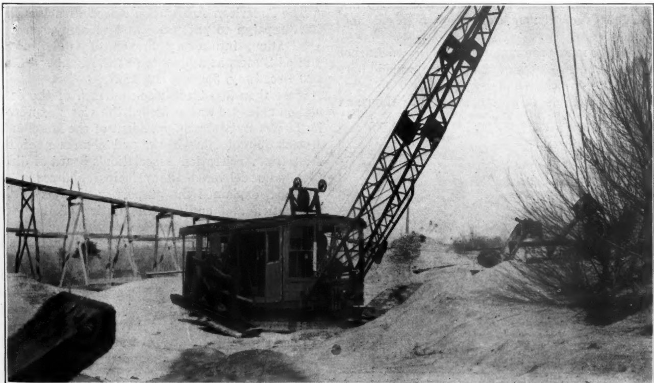
Walking Crane Used for Loading Trucks and Making Piles of Surplus
